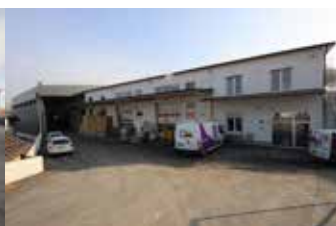
Compressors and technique dept. Service centre Welding department Dryers production Land: 31.500 m 2 Facilities: 4.100 m 2
