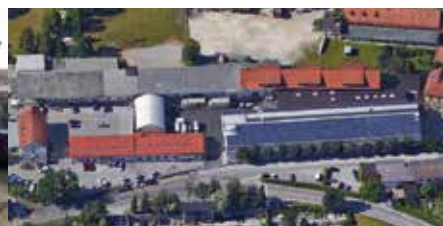
Head office Production halls Sales office R & D Area: 6.600 m 2
